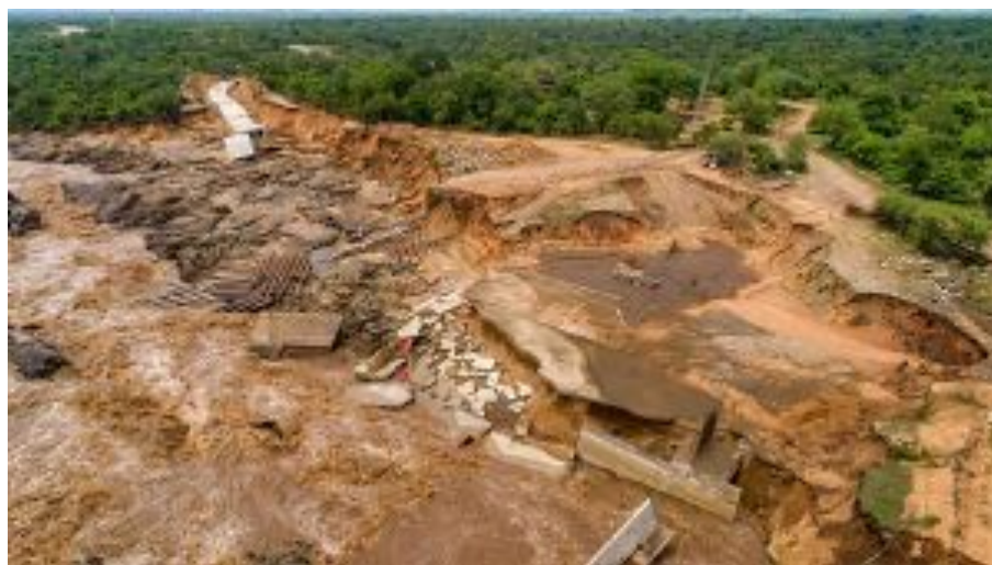
Figure 1-1: Kapichira Hydro-power plant damaged by Cyclone Ana in January 2022
